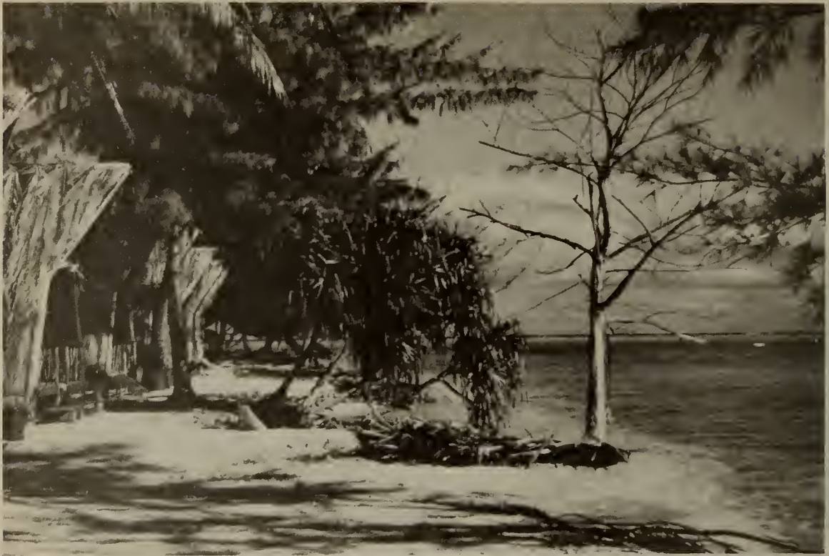
Fig. 37 Onetahi Islet, badly eroded beach front along passage; buildings were in use. MHS, 1982
