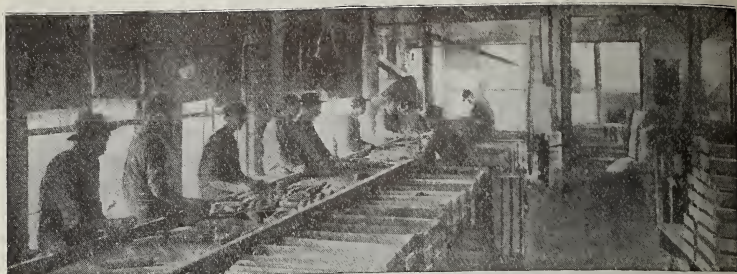
Inspecting and Sorting the Corn as It Passes Along a Wide and Slowly Moving Belt Before Going Into the Dry Kilns.
