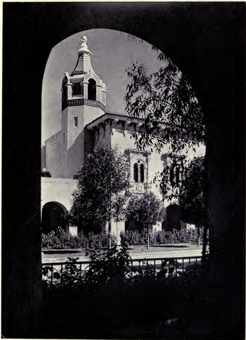
TOWER, AND PART OF SOUTH FACADE, SCIENCE AND EDUCATION BUILDING
