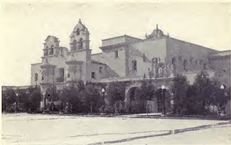
EAST FACADE, RUSSIA AND BRAZIL, BUILDING
