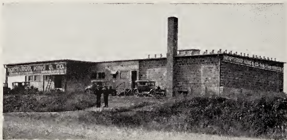
Northrup, King & Co. Country Drying Plant in West Central Minnesota
