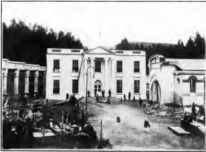
BUILDING OF THE UNITED STATES OF AMERICA, NEARING COMPLETION.
