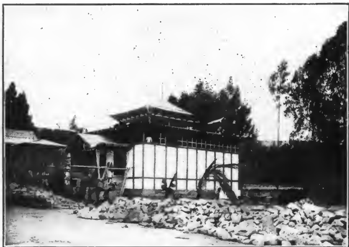
JAPANESE KIOSKS IN PROCESS OF CONSTRUCTION.
