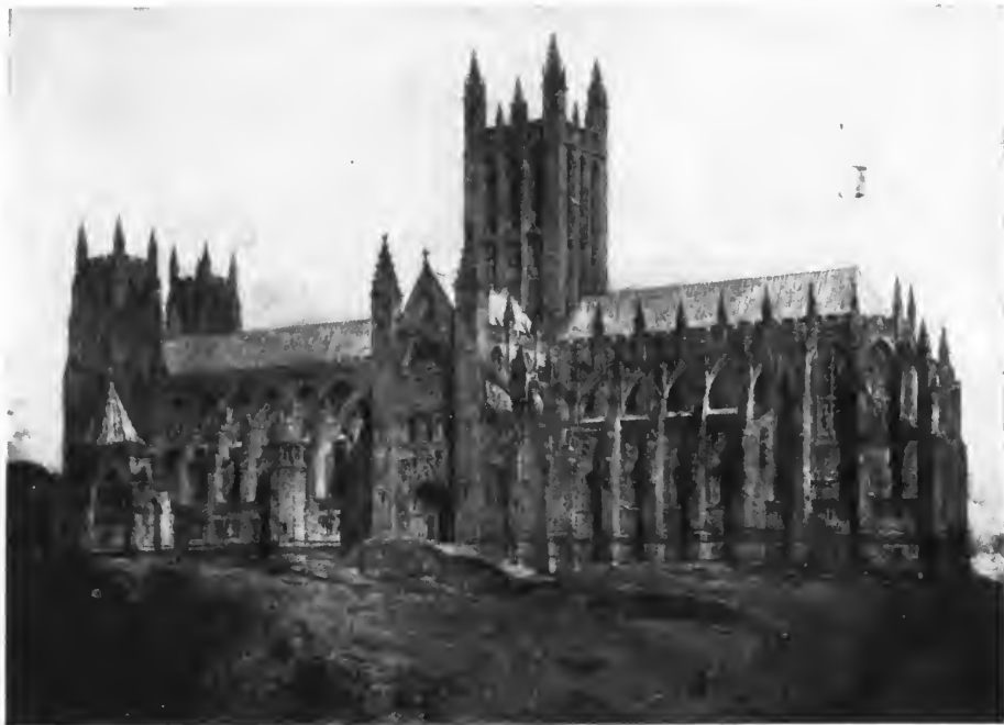
CATHEDRAL CHURCH OF ST. PETER AND ST. PAUL, WASHINGTON, DISTRICT OF COLUMBIA (FROM THE ARCHITECT'S DRAWING).
