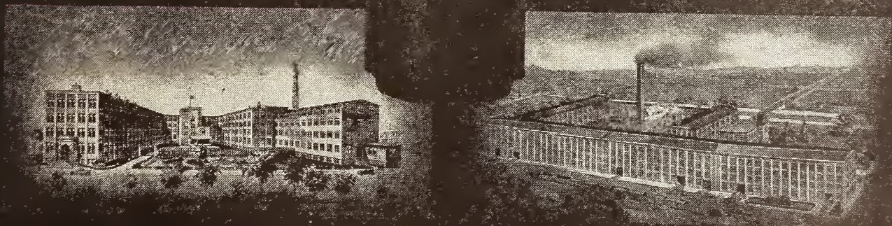
The Plant Behind It
