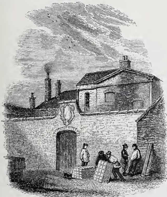
THE OVERHOUSE WORKS.
