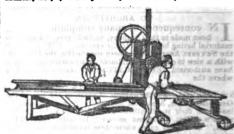
This is the most efficient Machine that has been invested for the purpose of making Drain Tiles. Any shaped This can be made by merely changing the die, which can be done in a few minutes. It requires but few hands, vin., one man and three boys. With this amount of labour, the pre-duct of a day of 10 hours is as follows, viz :---
