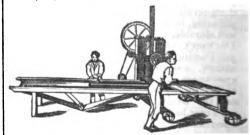
This is the most efficient Machine that has been invented for the purpose of making Drain Tiles. Any shaped Tile can be made by merely changing the die, which can be done in a few minutes. It requires but few hands, vis., one man and three boys. With this amount of labour, the pro-duct of a day of 10 hours is as follows, viz:--
