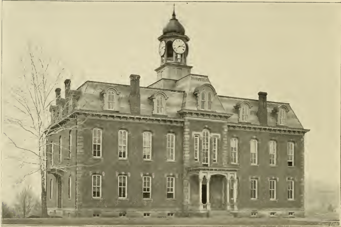
PREPARATORY BUILDING AND LIBRARY.
