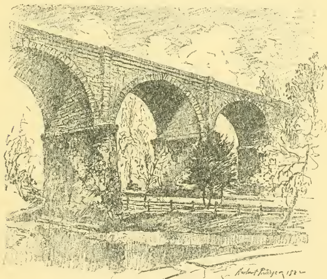
Railroad Bridge, Ridge Avenue Entrance
