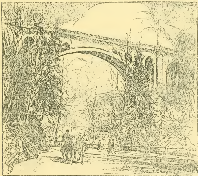
Walnut Lane Bridge
