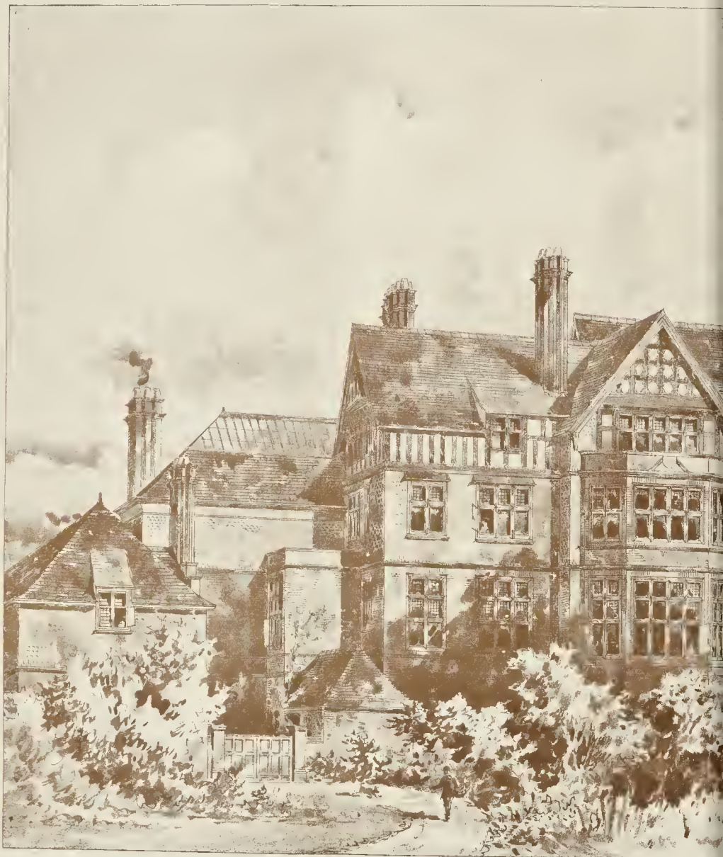
HATCHFORD, SURREY: VIEW OF ENTRANCE FRONT.
