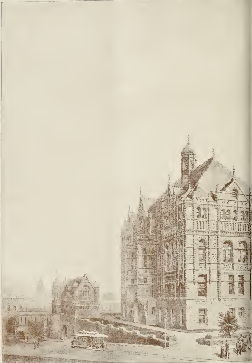
COURT HOUSE, LOS ANGELES COUNTY, CALIF.
