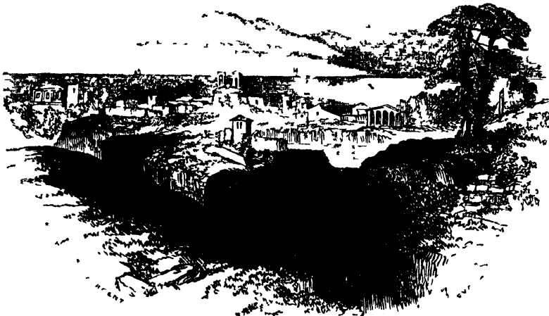
Fissures at Pollstena.
