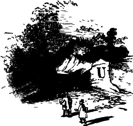
Flag Dyke, Brockhill Worcester
