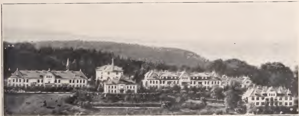
(Fig. 1). The Municipal Hospital, Lucerne, Switzerland
