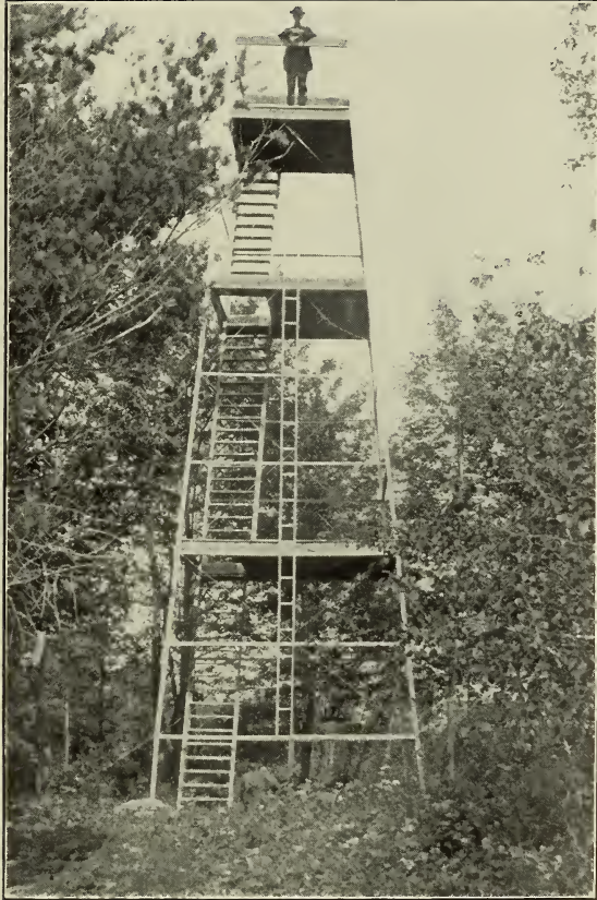
Steel tower (45 feet high) on Twadell Point Observ- vation Station, East Branch, N. Y.
