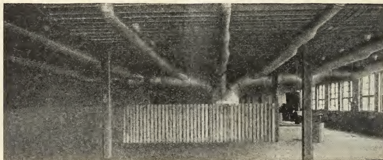
Large Conveyors Through Which Warm, Dry Air is Forced Into the Dry Kilns by a 13-foot Fan
