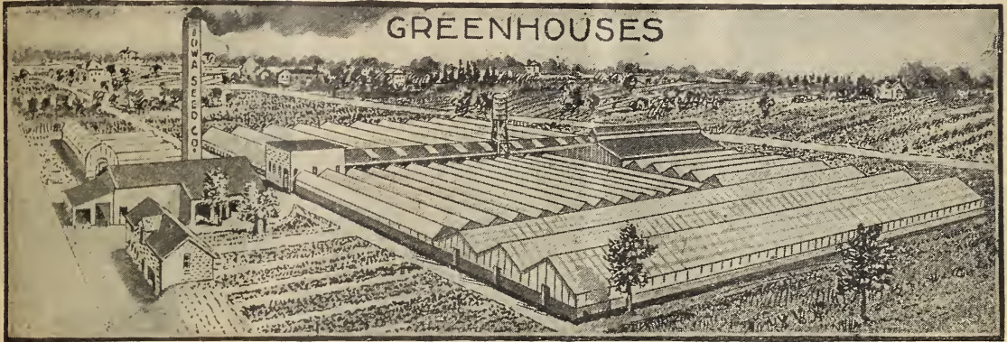
Iowa Seed Company's Thirty-two Greenhouses
