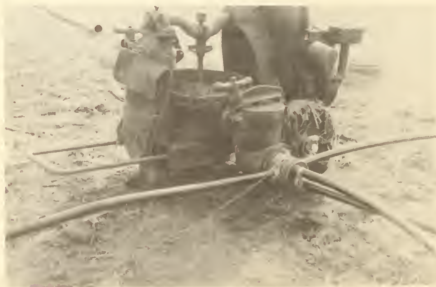
Figure 15.--Sump pump with connections.
