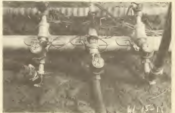
Figure 4.--Solenoid bank.
