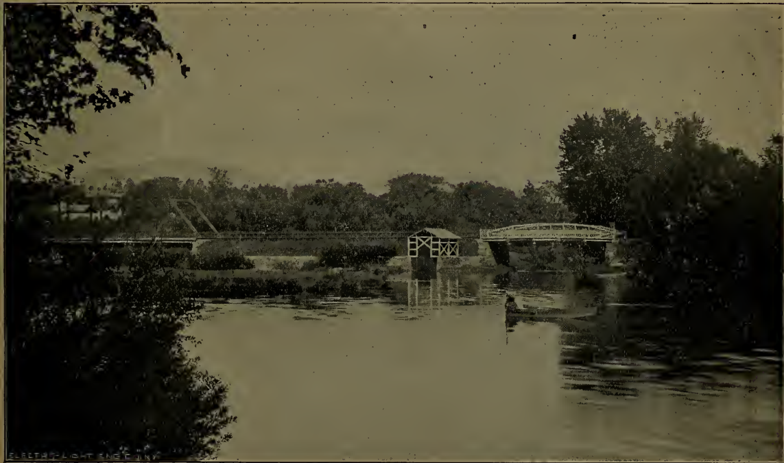
KINGSION STREET BRIDGE, DELHI.
