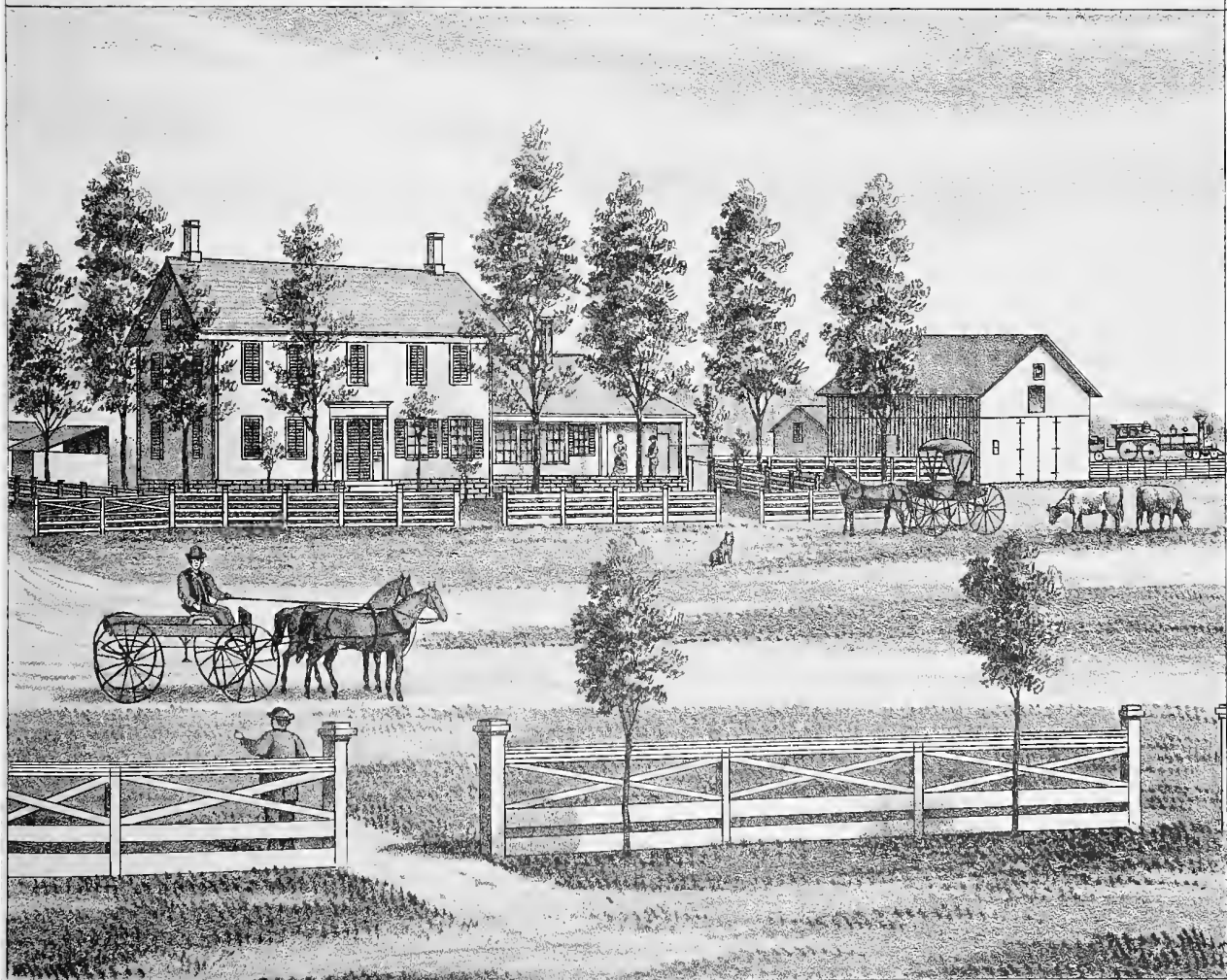
RESIDENCE OF IRA HALE, NORTH STOCKHOLM, ST. LAWRENCE CO., N.Y.
