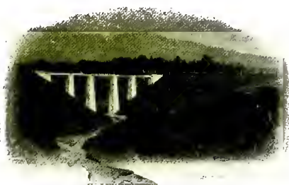
One of the Many Viaducts on the Government Railroad to Bandoeng.
