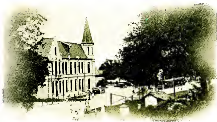
A Corner View of the K.P.M. Office.
