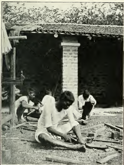
CARPENTERS AT WORK (p. 134)
