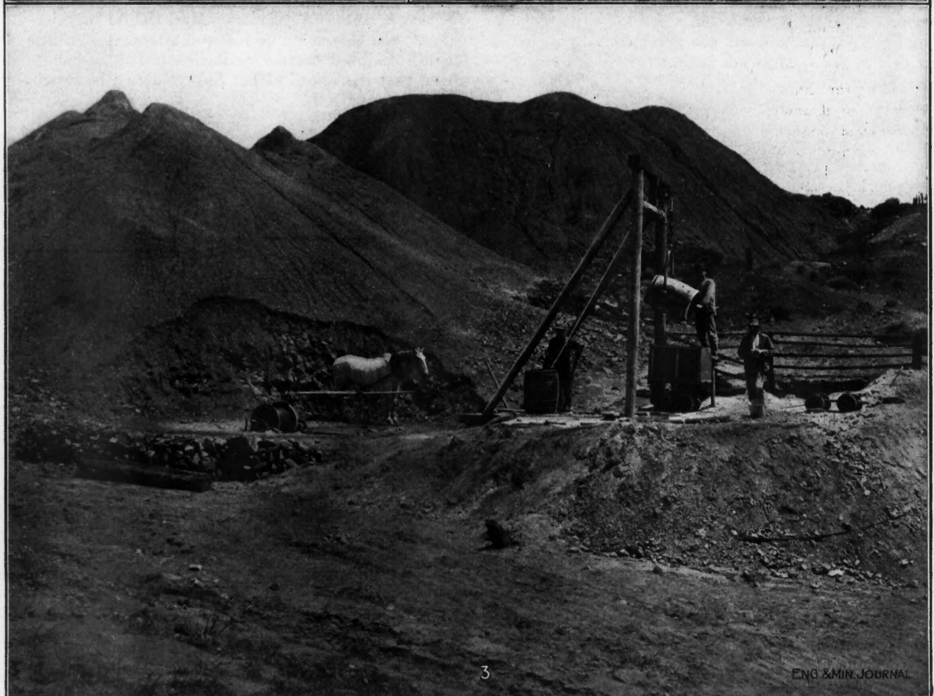
THE WAY SHAFTS ARE STARTED AT BUTTE, MONT.
