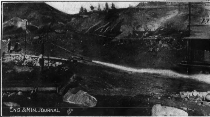
STRIPPING THE ROWE MINE, RIVERTON, MINN., CUYUNA IRON RANGE Hydraulic system used for removing overburden.
