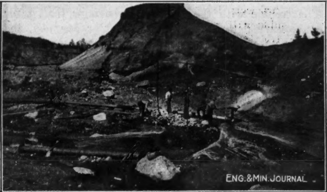
STRIPPING THE ROWE MINE, RIVERTON, MINN., CUYUNA IRON RANGE Hydraulic system used for removing overburden.
