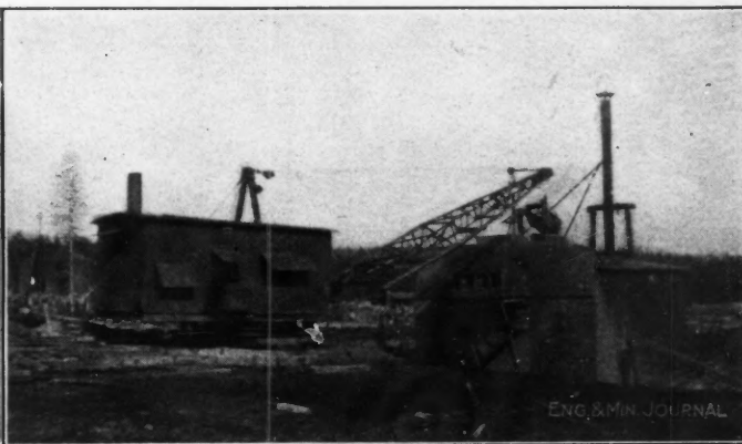
DRAG-LINE EXCAVATOR AND FLOATING WASHING PLANT
