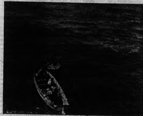
BUOYING THE CABLE.
