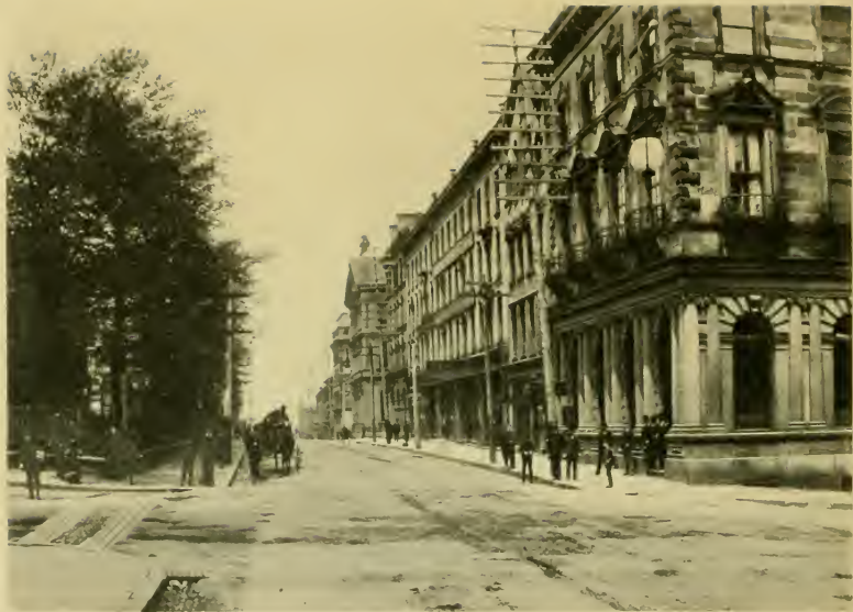
HOLLIS ST. LOOKING NORTH FROM PRINCE ST.
