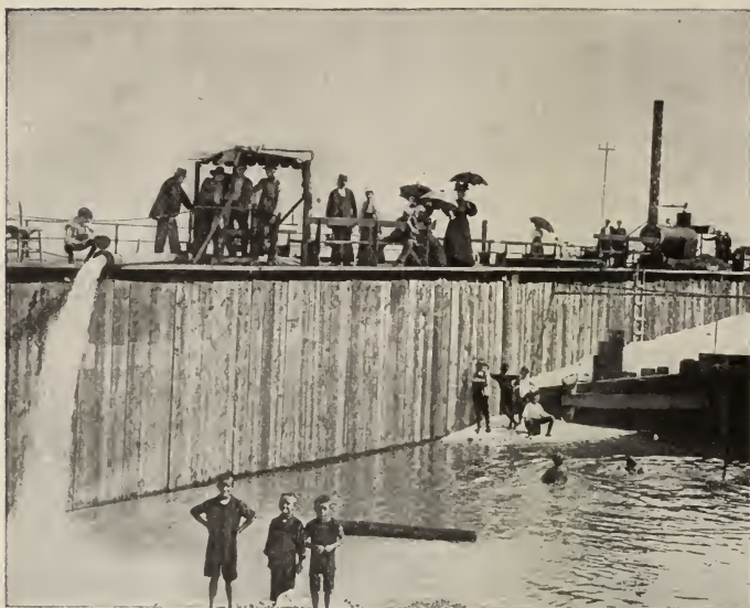
Filling Washout, July and August, 1896.
