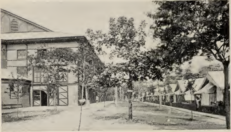
NEW AUDITORIUM. North Side—Showing Line of Tents.
