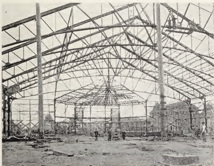
All the Main Trusses, Seven in Number, in position.
