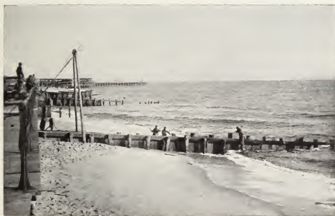
Building the Jetties.
