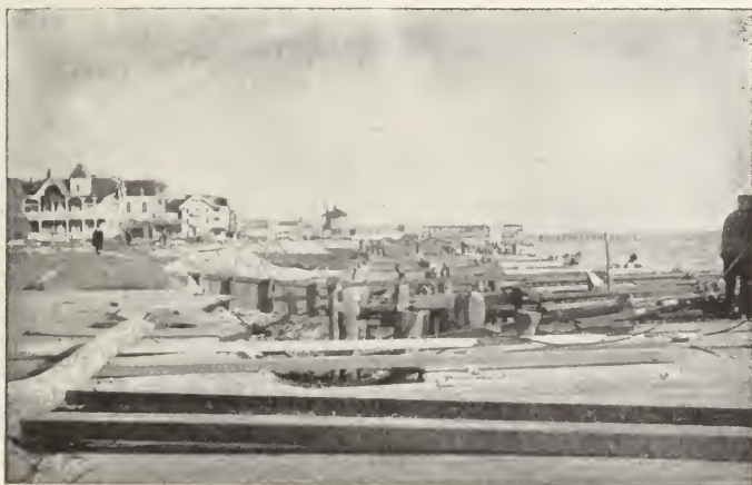
After the Storm of January 24, 1895. Preparing for Repairs.
