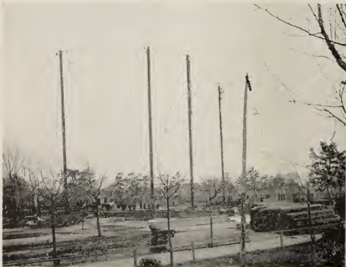
Masts in Position for erecting New Auditorium.
