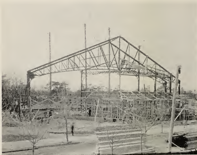
Two Main Trusses, also Angle Trusses in Position.
