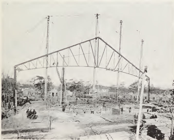
First Iron Truss in Place.
