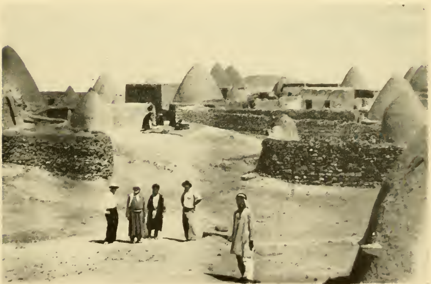
2. GENERAL VIEW OF A "BEEHIVE" VILLAGE IN THE ALLOUITE REGION, NORTH SYRIA.
