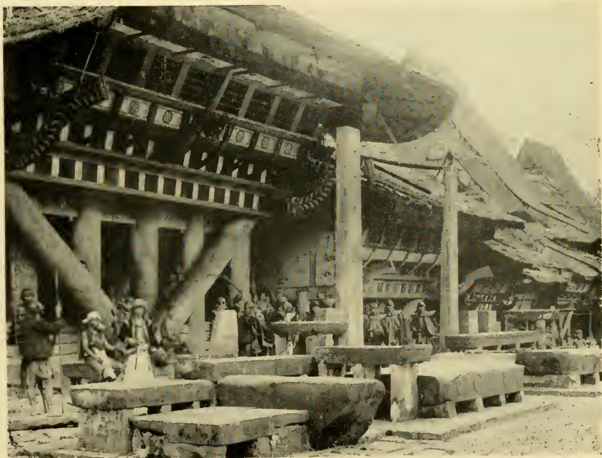
2. HOUSES IN NIAS WITH MASSIVE TIMBERS, CARVED AND PAINTED GABLES, AND HOODED ROOFS.
