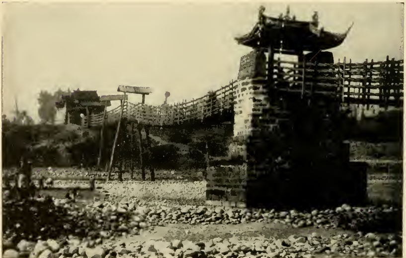
2. CHINESE SUSPENSION BRIDGE WITH BAMBOO CABLES.
