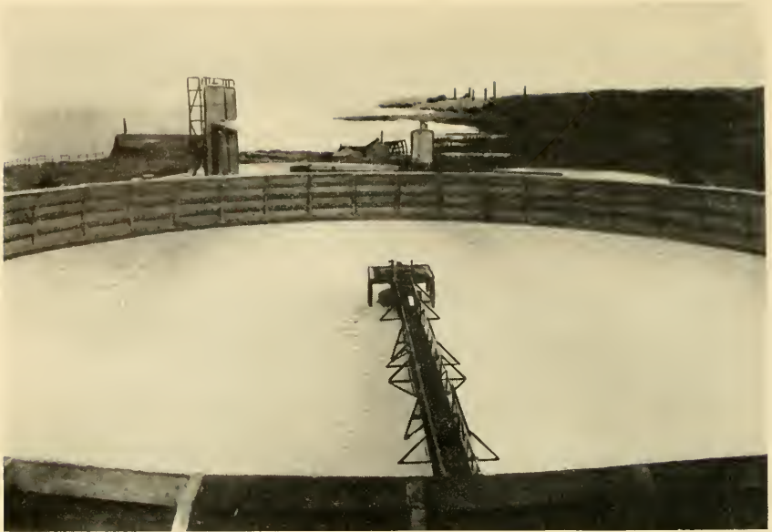
1. SETTLING TANK, WHICH HAS A CAPACITY OF 2,000,000 GALLONS OF WATER AND APPROXIMATELY 1,000 TONS OF MAGNESIUM HYDROXIDE.
