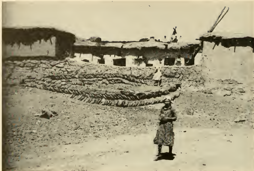
1. TYPICAL HOUSE IN THE BIKA' PLAIN, LEBANON.
