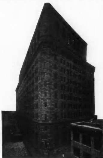
Federal Reserve Bank of New York York and Sawyer, Architects
