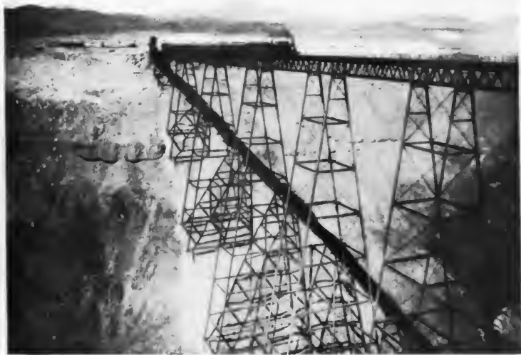
A VIADUCT ON THE ANTOFAGASTA-BOLIVIA RAILWAY
