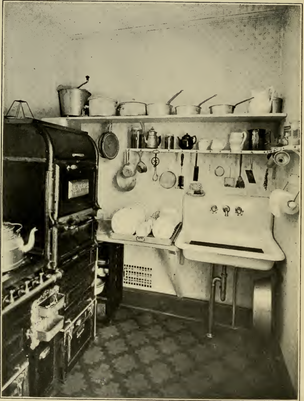
KITCHENETTE WITH GAS-RANGE.
