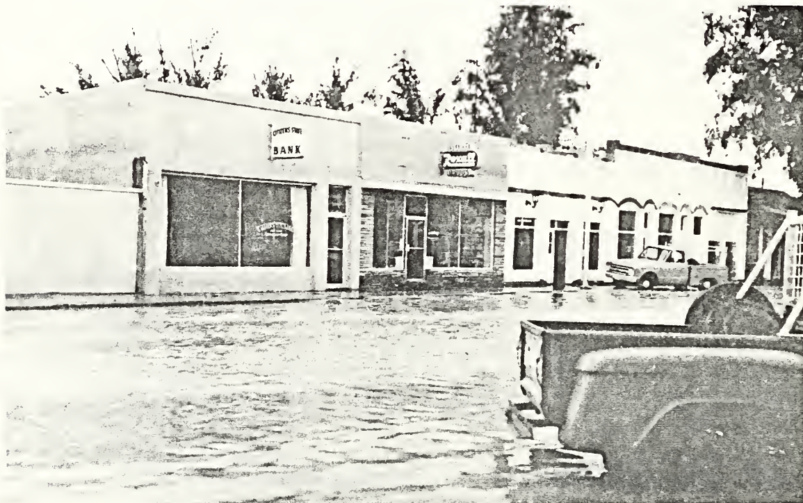
Main street of Estancia, New Mexico under floodwaters from Milbourne and Compton Draws
