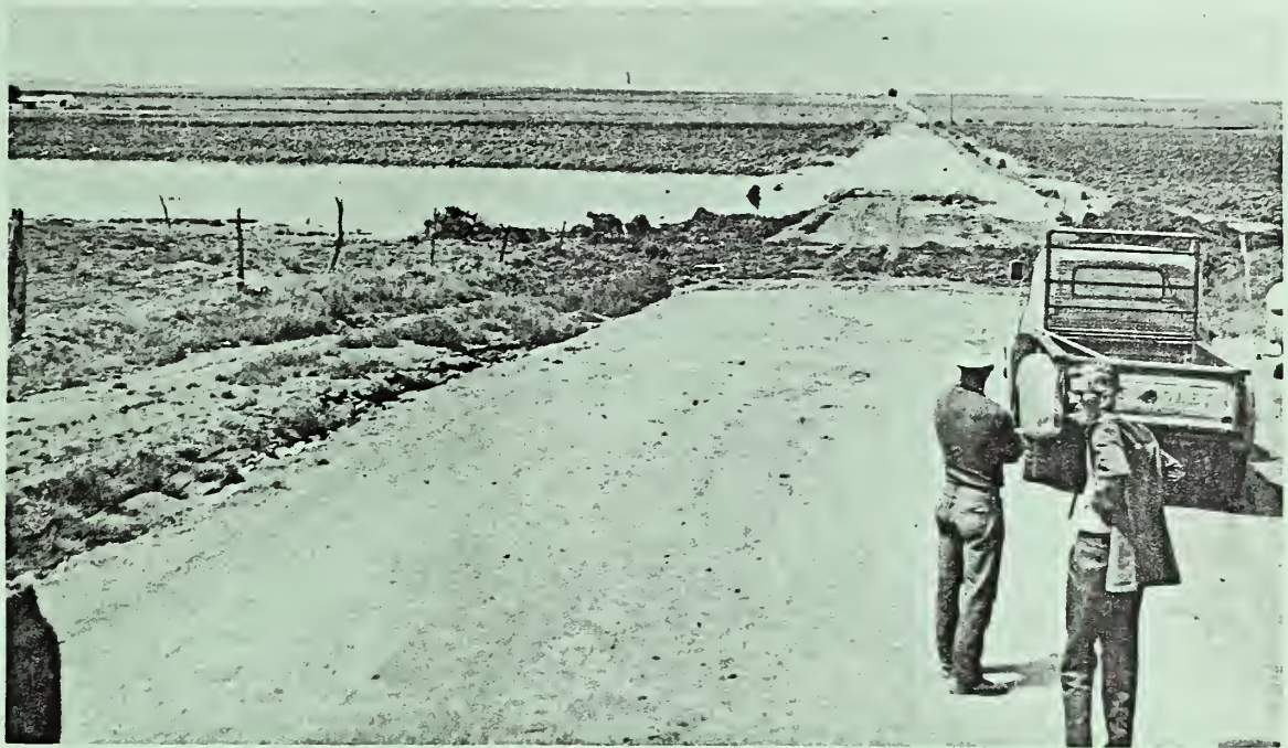
Flood damage to roads and crops
