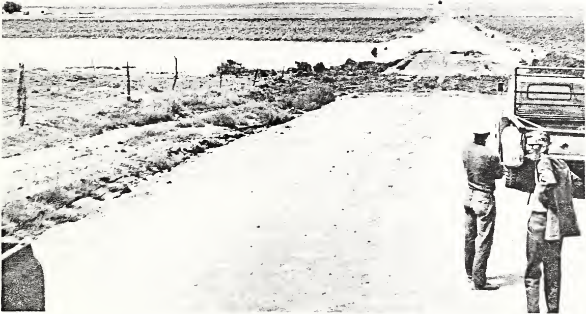
Highway and crop damage from floodwater from Tajique and Torreon Draws.
