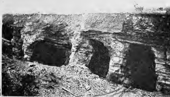
WORKINGS AT HOLLYWOOD COLLIERY NO. 1. - LOOKING SOUTH (PICTURE REVERSED.)
