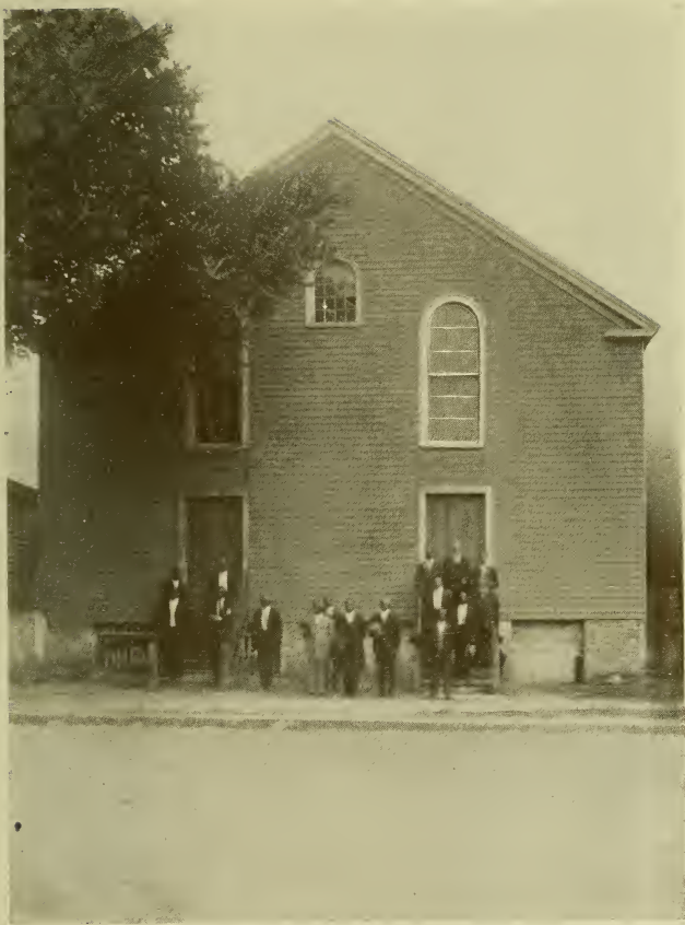
SPRINGFIELD BAPTIST CHURCH, AUGUSTA, GA. (Old Building)
