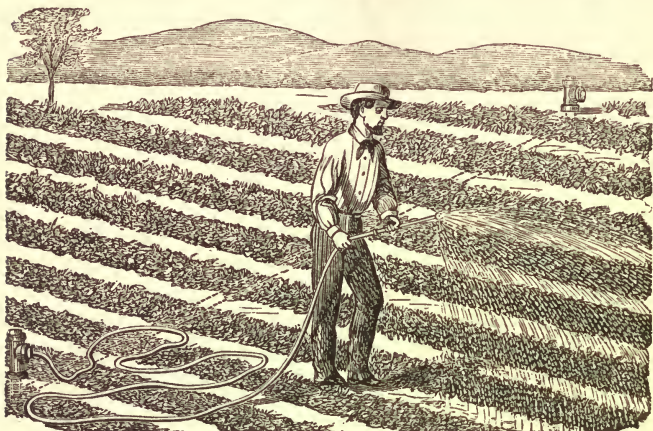
Fig. 21.—IRRIGATING BY PIPES AND HOSE.
