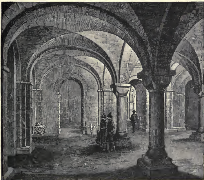
CRYPT IN BOW CHURCH, FROM THE NORTH SIDE, NEAR THE EAST END OF THE NAVE
