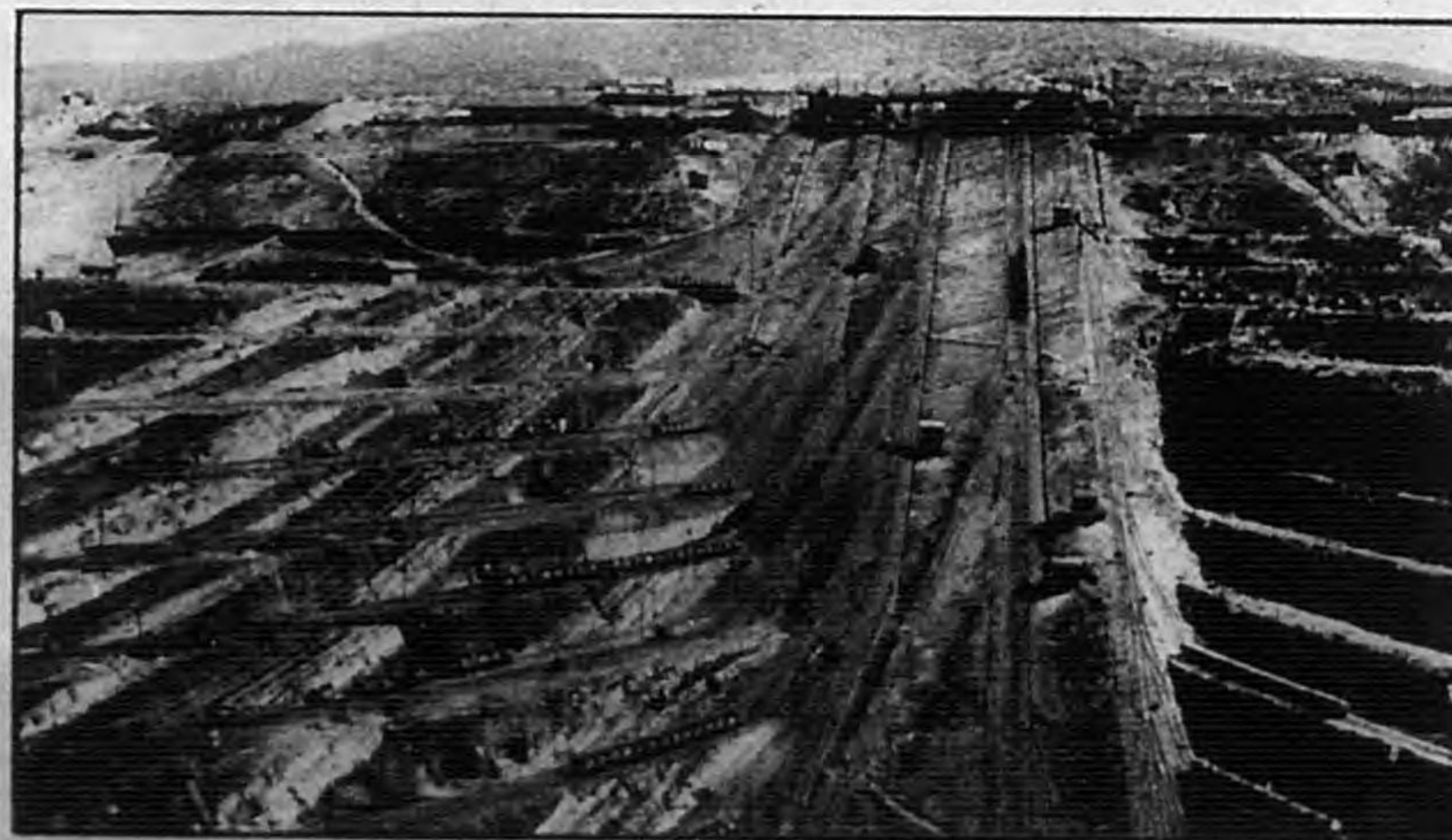
The Open Cut at Fushum Colliery
