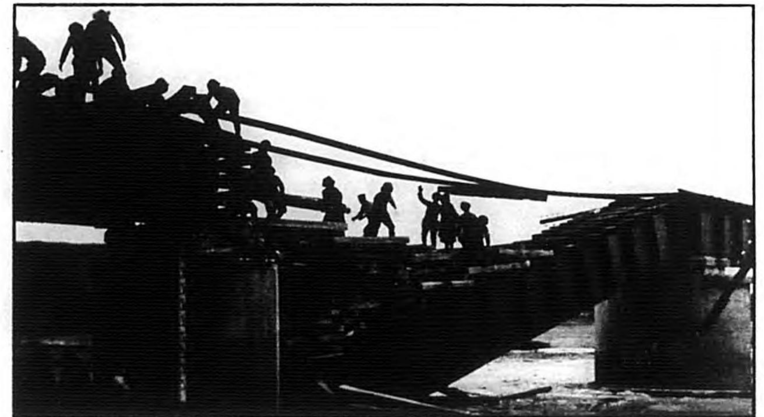
Japanese Troops Repairing Railway Bridge Destroyed by Chang Hsueh-liang's Soldiers (Hsiaoling River on the Mukden-Shanhaikwan Line)
