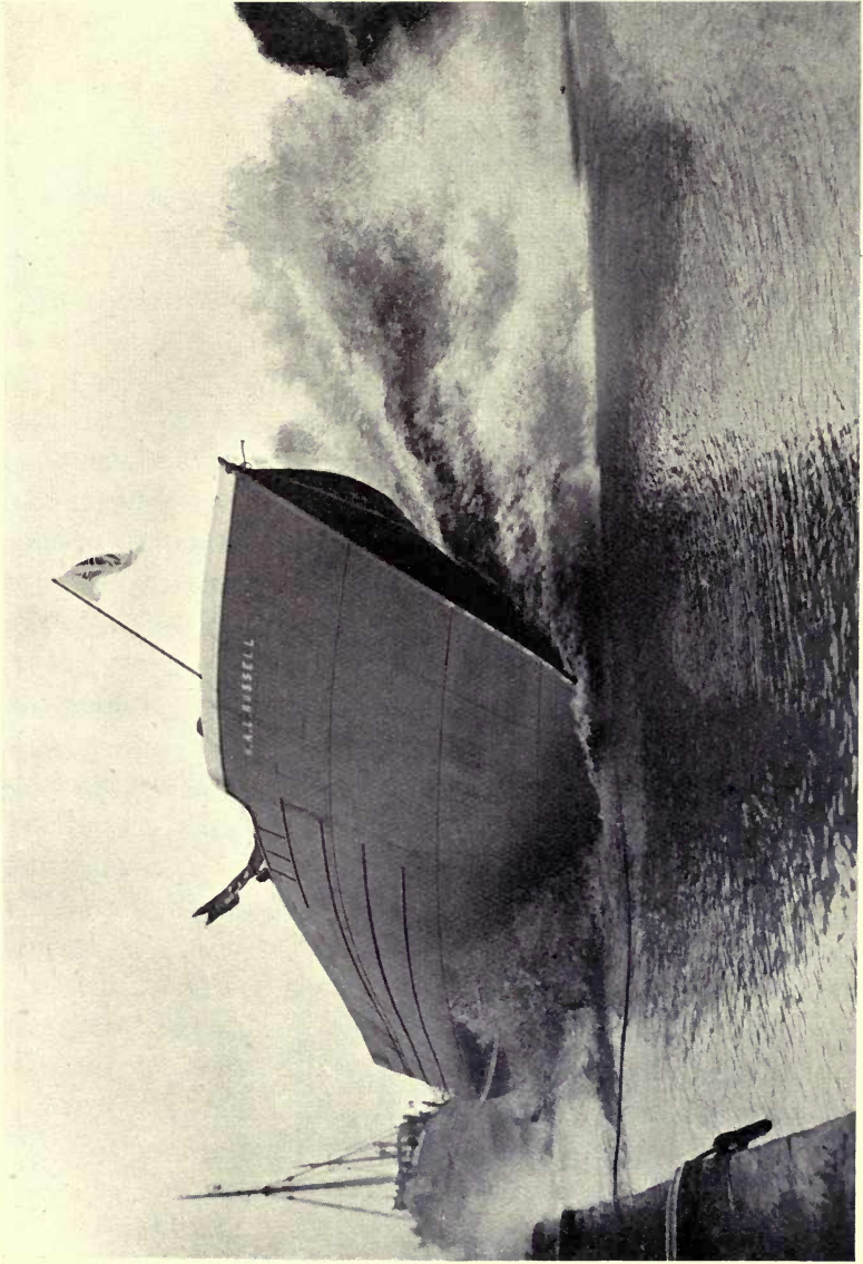
LAUNCHING A STEAM-TRAWLER, BROADSIDE ON, AT THE YARD OF MESSRS. COCHRANE, SELBY, YORKS.
