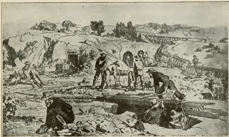
DIGGING AND WASHING GOLD
