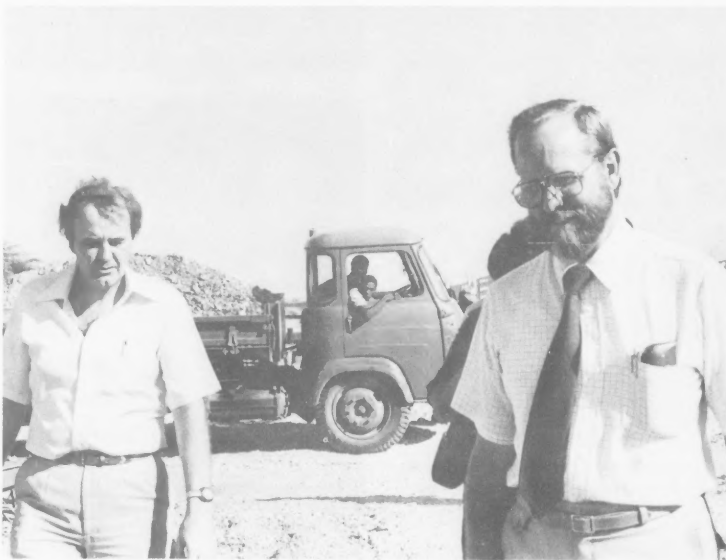
At warehouse construction site are Paul Hartenberger , an AID project manager, and Jerry Russell , chief public health officer.
