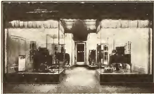
Exterior of New Brunswick Shop
