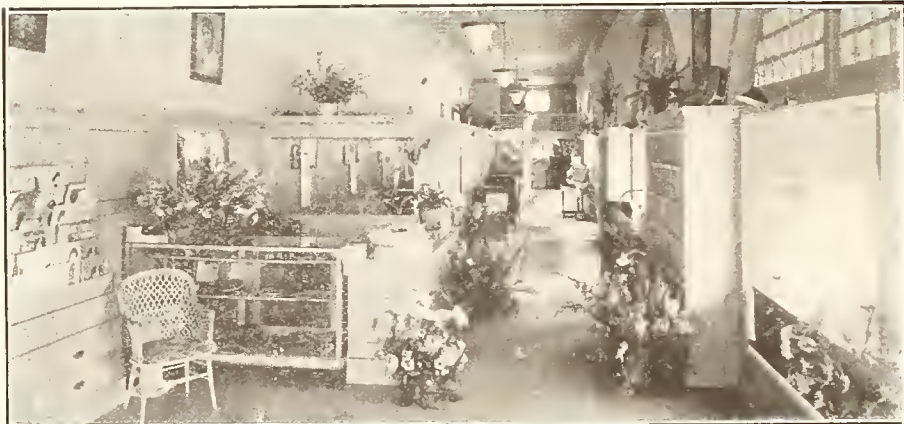
Interior View of Don C. Preston's New Store
