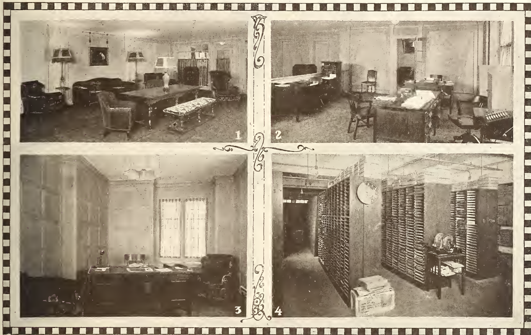
Views of New Home of Ormes, Inc. 1—Reception Foyer. 2—General Offices. 3—C. L. Price's Private Office. 4—View of Record Vaults
