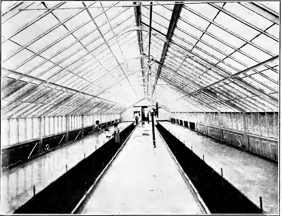
Sub-Irrigation Benches Testing the Cement Tanks for leaks
