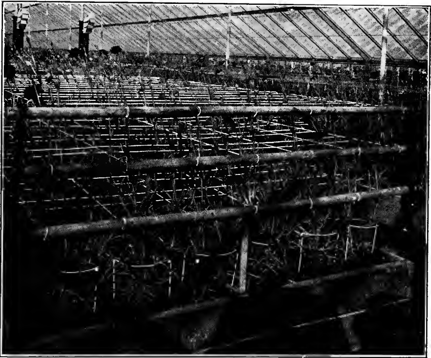
Illustrating End Supports of Iron for Stretching Wire
