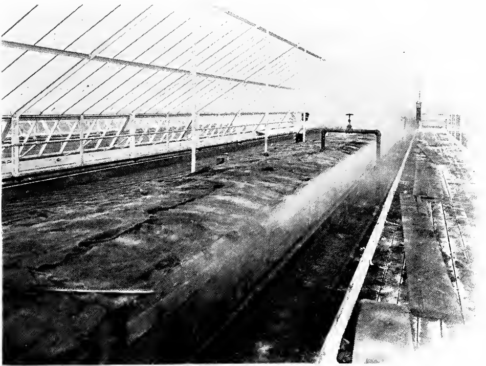
Soil Sterilizer in operation—Sterilizing soil on the bench
