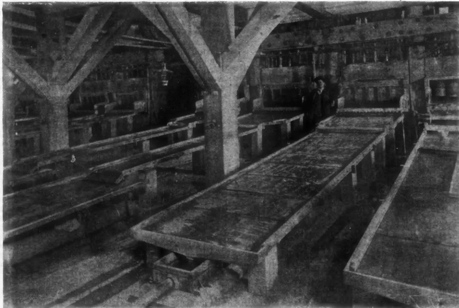
NORTH STAR MILL, AMADOR COUNTY, CAL.
