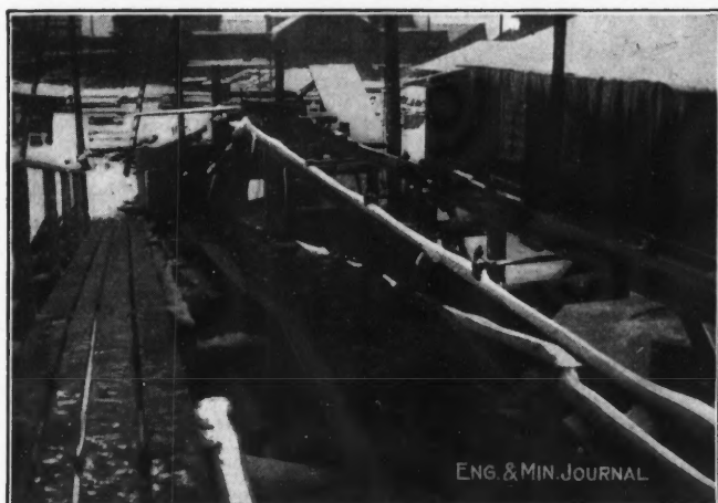
STEEL-BELT CONVEYOR HANDLING BROKEN AND LUMP MATERIAL
