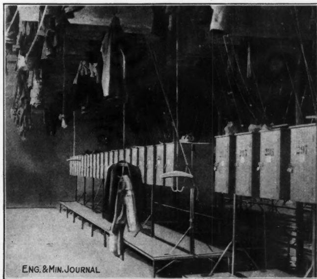
FIG. 2. INSIDE OF CHANGE HOUSE, SHOWING SMALL LOCKERS AND CLOTHES SUSPENDED FROM HOOKS
