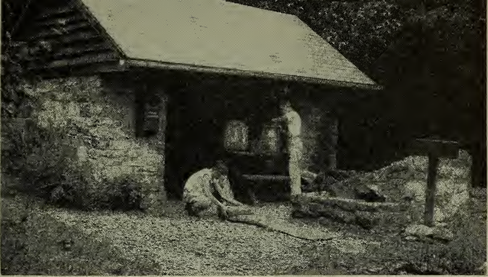
The lean-tos of the early Appalachian trail have changed. Now they are elaborate and roomy like this well-protected building.
