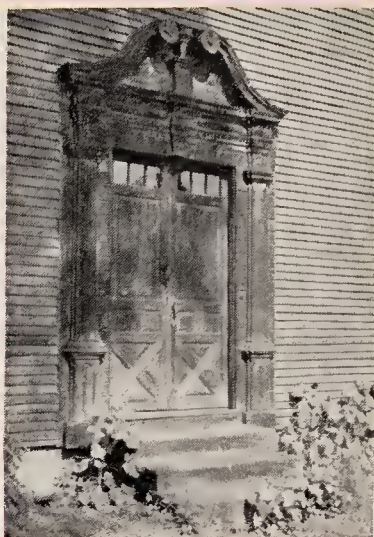
Door of the Reverend John Williams' house, Old Deerfield, Mass., built in 1707.
