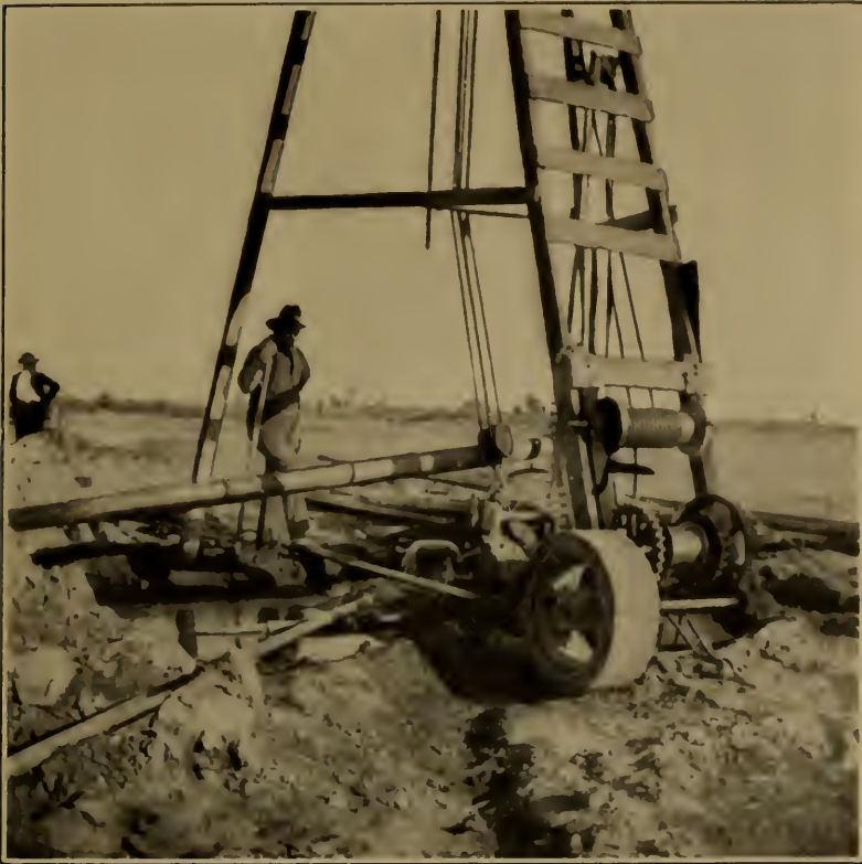
A. TYPE OF WELL-DRILLING RIG USED IN ANTELOPE VALLEY.
