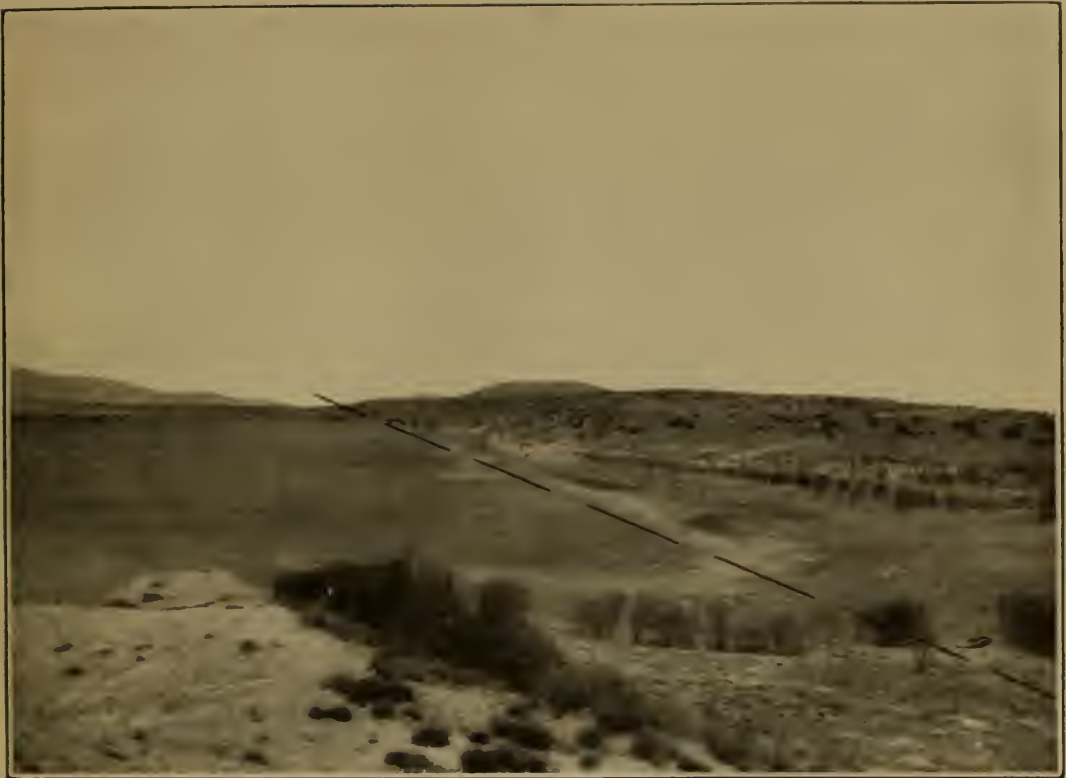
A. PALMDALE RESERVOIR, LOOKING NORTHWEST.
