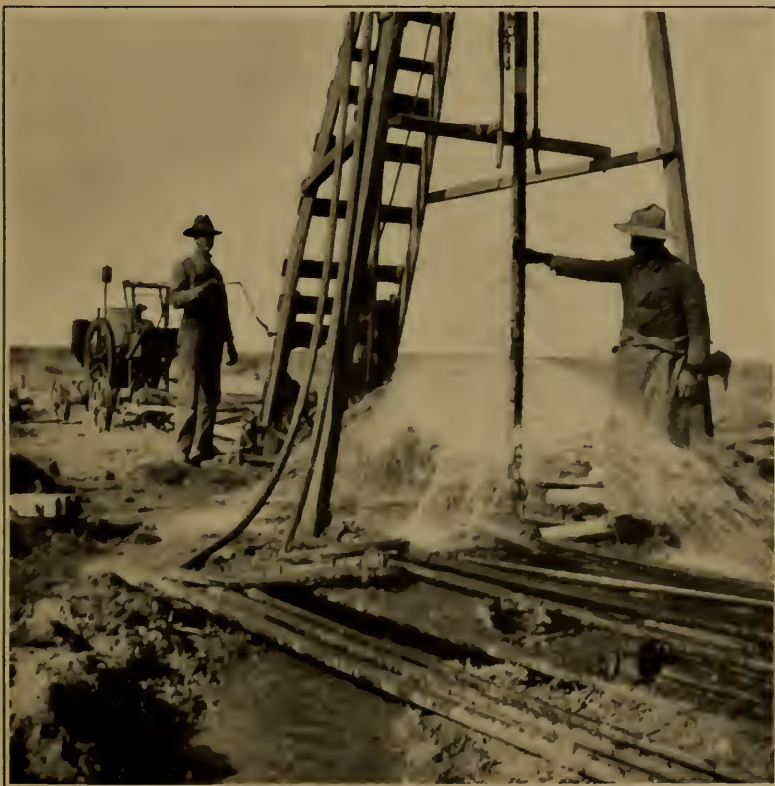
B. INSERTING PERFORATED CASING IN PARTLY COMPLETED ARTESIAN WELL.
