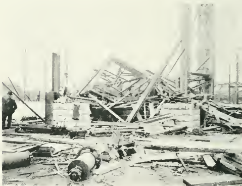
COLLAPSE OF SCOTCH CRANE ON NEW BUILDING SITE, SEPTEMBER 10TH, 1903.
