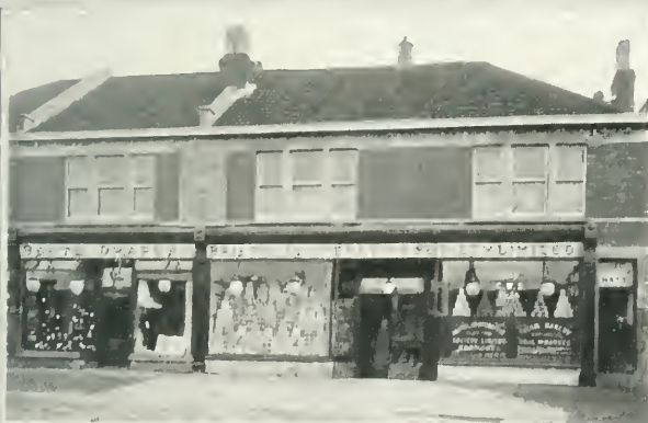
GLOUCESTER ROAD BRANCH, BISHOPSTON.
