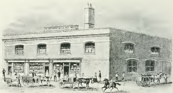
OLD KINGSLAND ROAD STORES.
