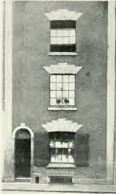
FIRST PREMISES, HOULTON STREET, 1884.
