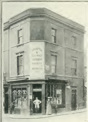
ST. GEORGE'S ROAD BRANCH, 1891.
