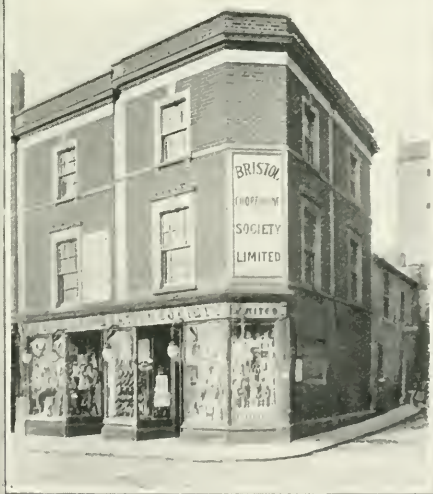
ST. GEORGE'S ROAD BRANCH, 1909
