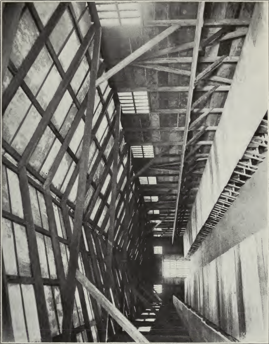
CONVICTS' CAMP, JAYUYA. INTERIOR OF BARRACKS.
