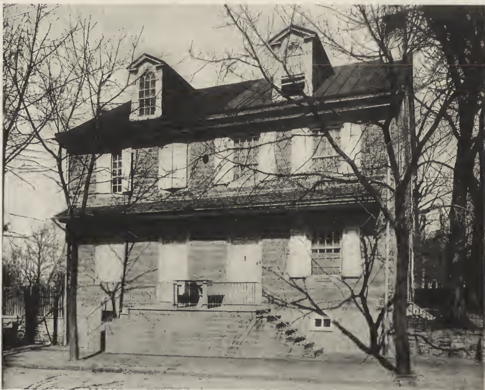
THE BILLMEYER HOUSE, GERMANTOWN, PA., SHOWING USE OF PENT-ROOF. 1727.
