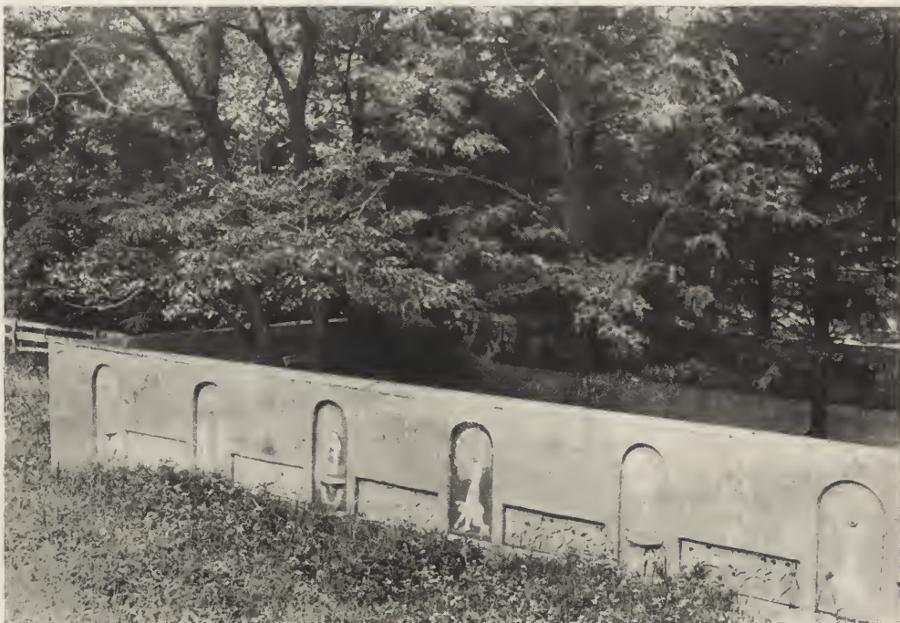
VIEW OF GARDEN FROM HILL ABOVE THE STUDIO, SHOWING POSITION OF LONG FRIEZE ON INNER WALL.
