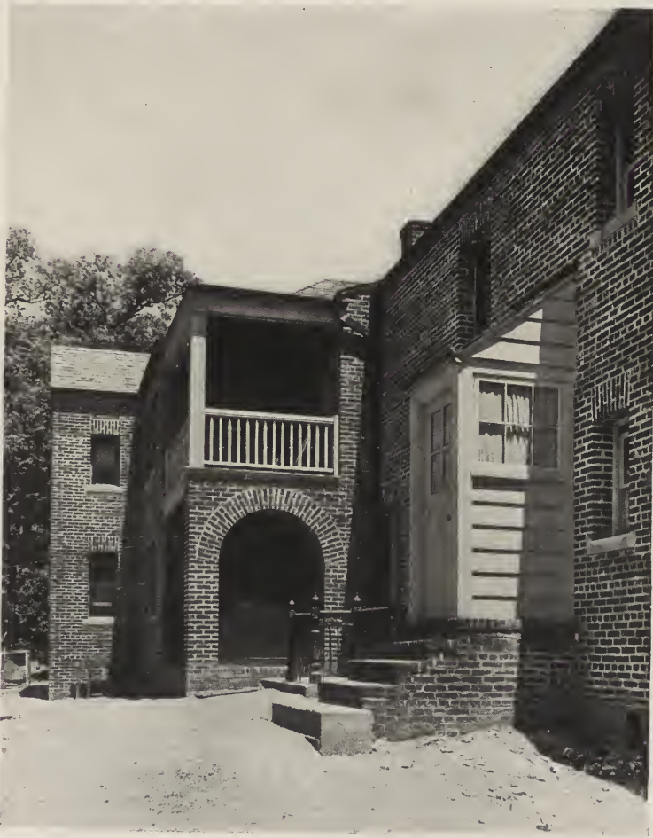
DETAIL OF GARDEN APARTMENT HOUSE IN BRONX BOROUGH, NEW YORK CITY. Clarence S. Stein, Architect.
