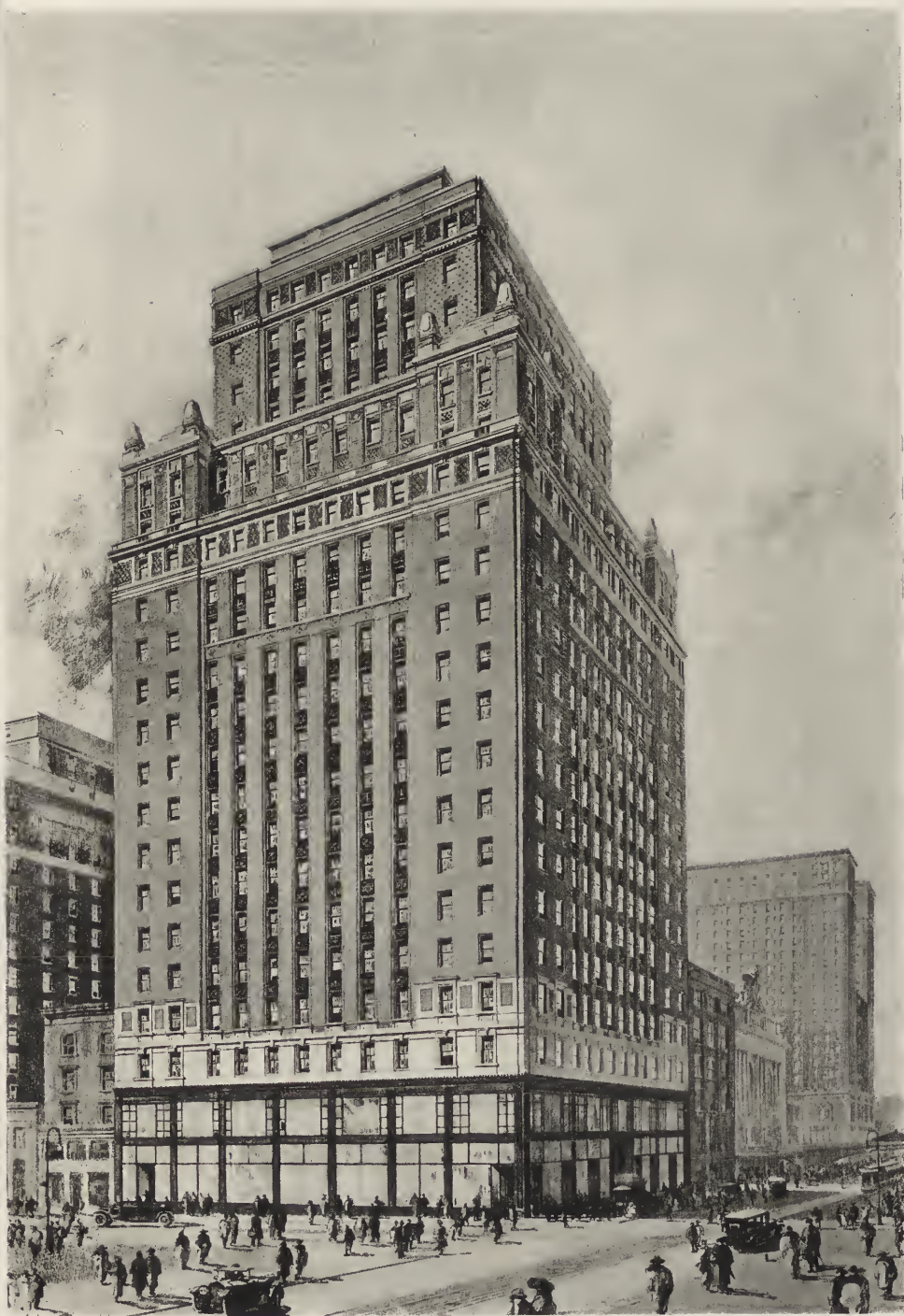
LIGGETT-WINCHESTER-LEY CORPORATION BUILDING, NEW YORK CITY. CARRÈRE & HASTINGS, AND R. H. SHREVE, CONSULTING ARCHITECTS.
