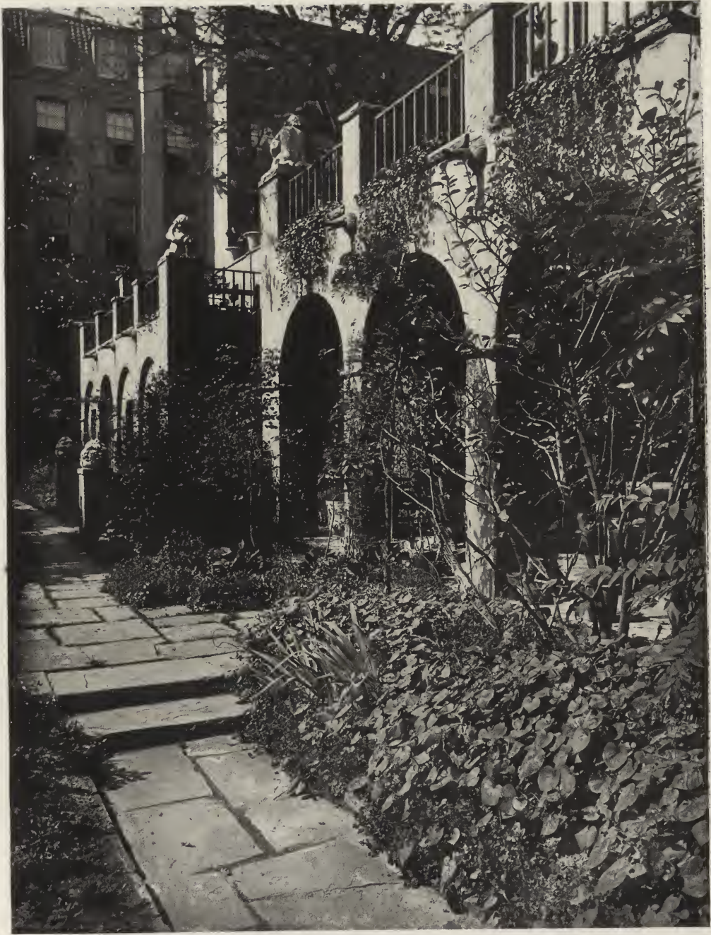
THE LOGGIA ARCHES IN THE WEST END OF THE GARDEN HAVE THE DECORATIVE EFFECT OF A ROMAN AQUEDUCT—TURTLE BAY GARDENS, NEW YORK CITY. EDWARD C. DEAN AND WILLIAM LAWRENCE BOTTOMLEY, ASSOCIATE ARCHITECTS.
