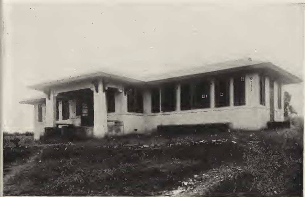
HONOR COTTAGE AT INSULAR REFORM SCHOOL, MAYAGUEZ, P. R., WHERE BOYS ARE HOUSED WHO MERIT DISTINCTION FOR GOOD CONDUCT.
