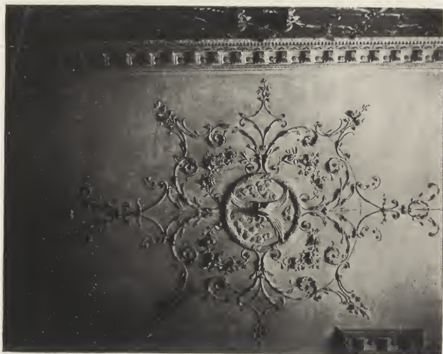
STAIRCASE CEILING—BEACON HOUSE, PAINSWICK, GLOUCESTER.
