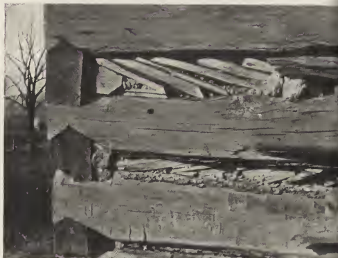
ANGLE VIEW OF EARLY LOG HOUSE, SHOWING "CHINKING."
