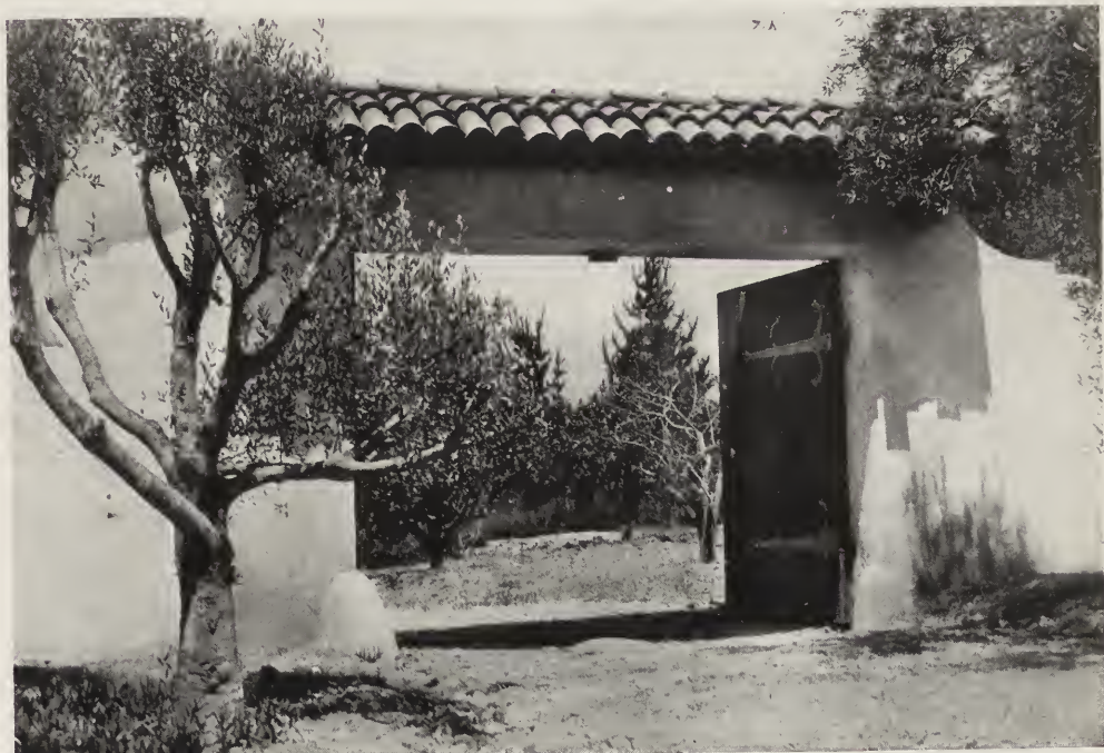
FARM GATE—RESIDENCE OF MRS. MARY E. STEWART, SANTA BARBARA, CAL. George Washington Smith, Architect.
