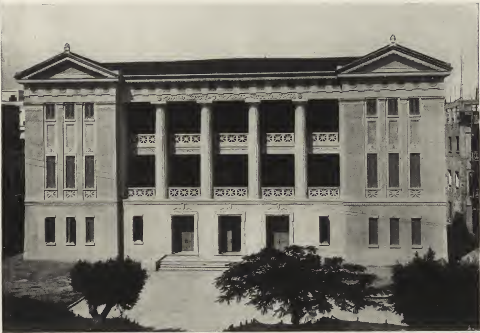
ROMAN BALDORIOTY DE CASTRO GRADED AND TECHNICAL SCHOOL, SAN JUAN, P. R.
