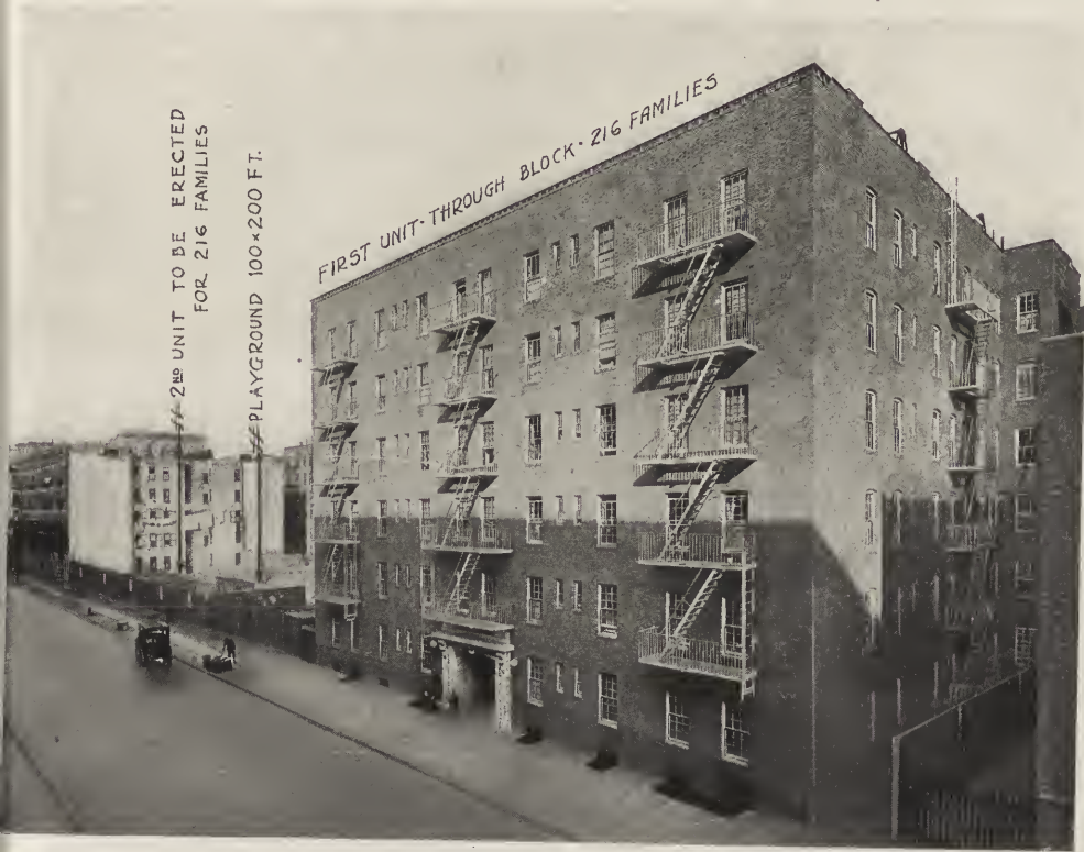
FIRST UNIT ERECTED—OPEN-STAIR APARTMENTS ON WEST 146th AND 147th STREETS, NEW YORK CITY.
