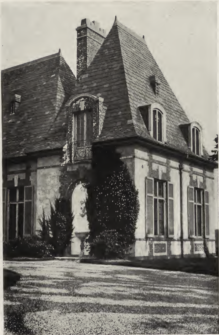
RESIDENCE AT WOODBURY, L. I., OF PHILIP L. GOODWIN, OF GOODWIN, BULLARD & WOOLSEY, ARCHITECTS.
