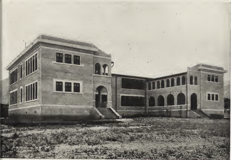
REAR VIEW—TWELVE-ROOM SCHOOL IN CAYEY, P. R.
