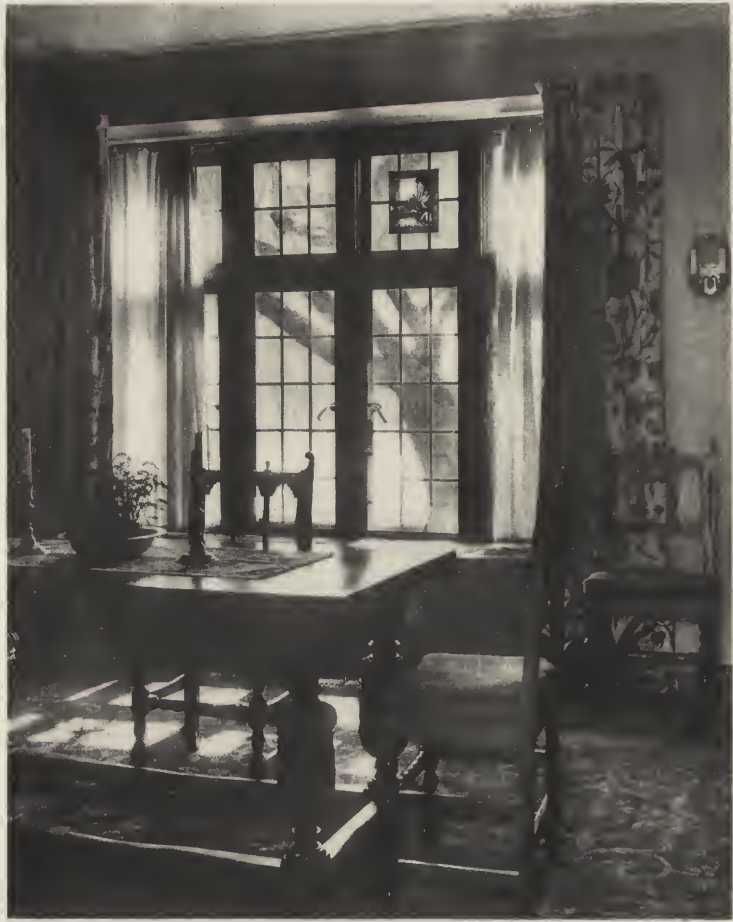
DETAIL OF DINING ROOM—RESIDENCE OF MRS. ARTHUR CAHN, HARTSDALE, N. Y. Alfred Hopkins, Architect.
