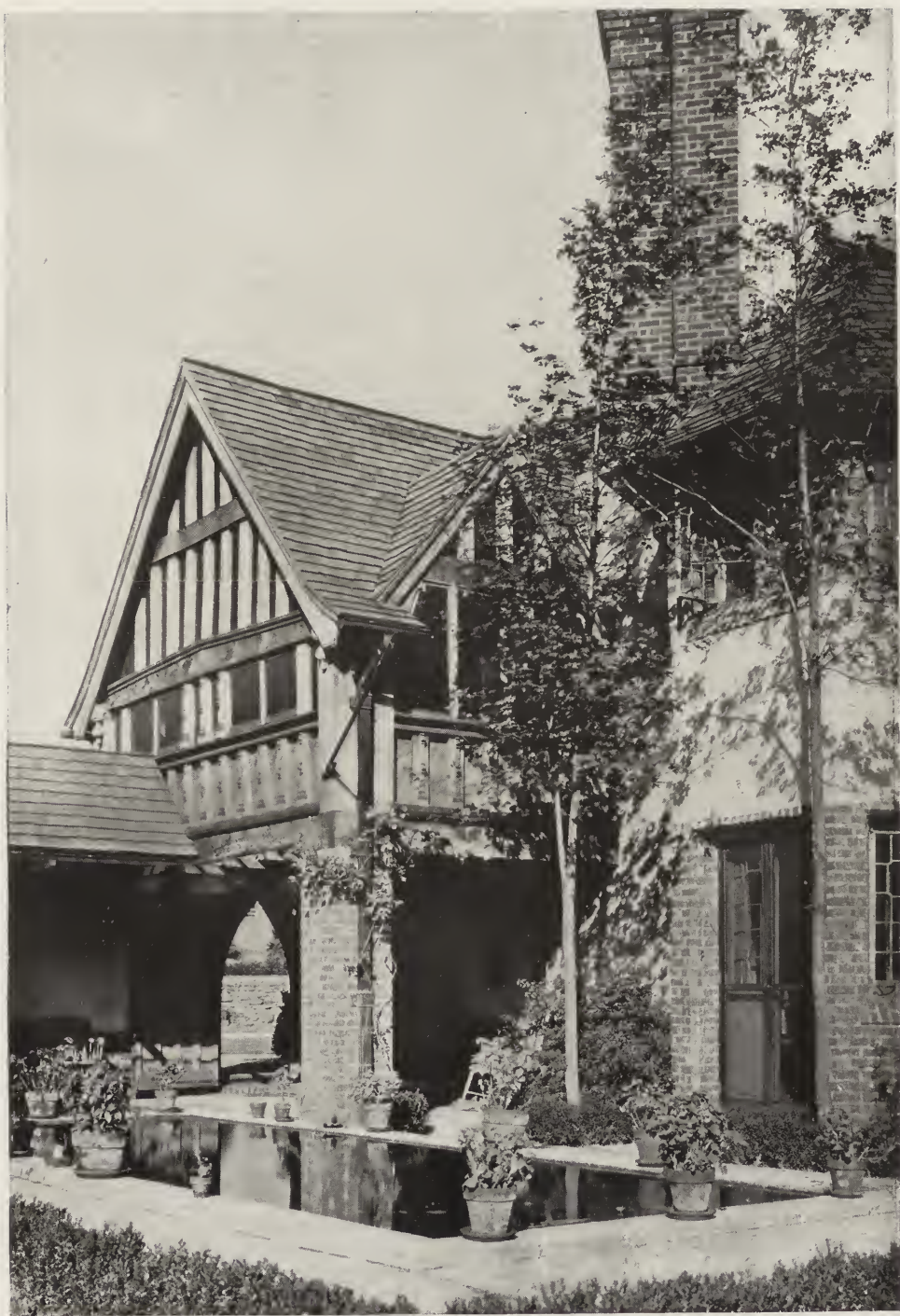
THE POOL AND THE SLEEPING PORCH—RESIDENCE OF CASPAR W. MORRIS, ESQ., HAVERFORD, PA. MELLOR, MEIGS & HOWE, ARCHITECTS.
