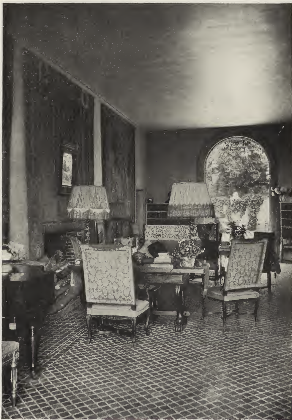
THE LIVING ROOM LOOKING TOWARD FORECOURT (POINT OF VIEW 9 ON PLAN)—RESIDENCE OF GEORGE HOWE, ESQ., CHESTNUT HILL, PHILADELPHIA. MELLOR, MEIGS & HOWE, ARCHITECTS.
