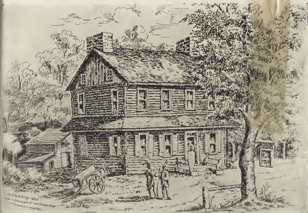
POSTLEWAITE'S TAVERN, NEAR LANCASTER, PA. EARLY USE OF PENT-ROOF. 1729.
