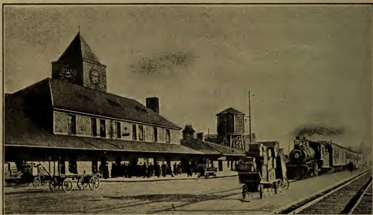
Great Northern Station
