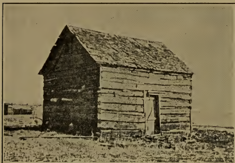
Poorly Ventilated House
