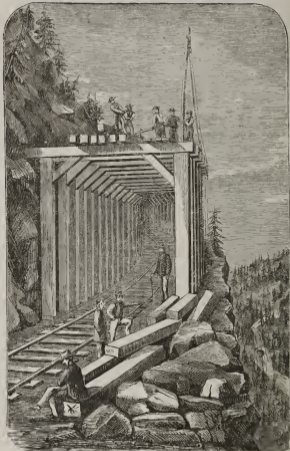
Constructing Snow Sheds, Sierra Nevada Mountains, C. P. R. R. See page 192.
